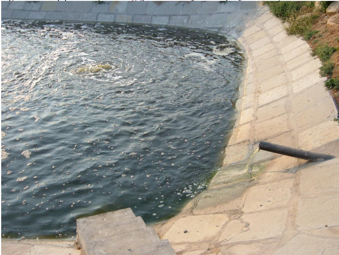
Figure 3. Northern Part of the Aeration Pond (Pond #2), showing the discharge from Pond #1 into it (Photo: Srikant, Dec 26, 2004)
